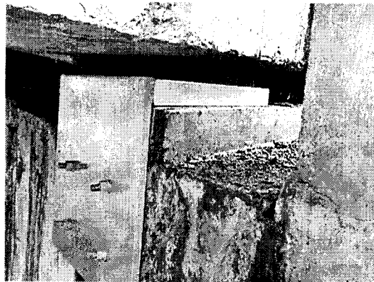
Figure 9 : Complete Installation and Fabrication of New Elastomeric Bearing Pad
